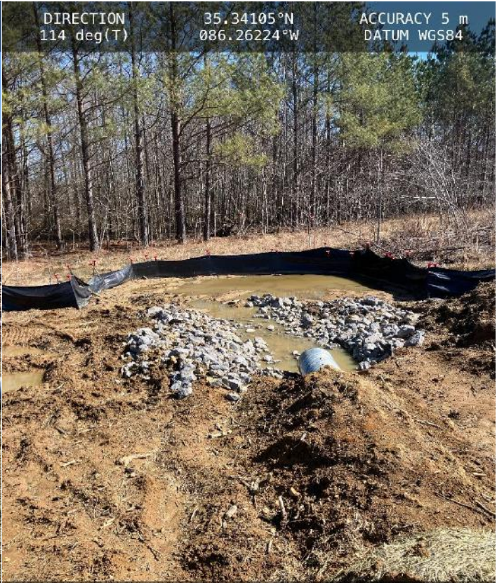
Zone 15 – Basin 35 Stabilize and Repair SF 2026-02-13 11:38:53-06:00
