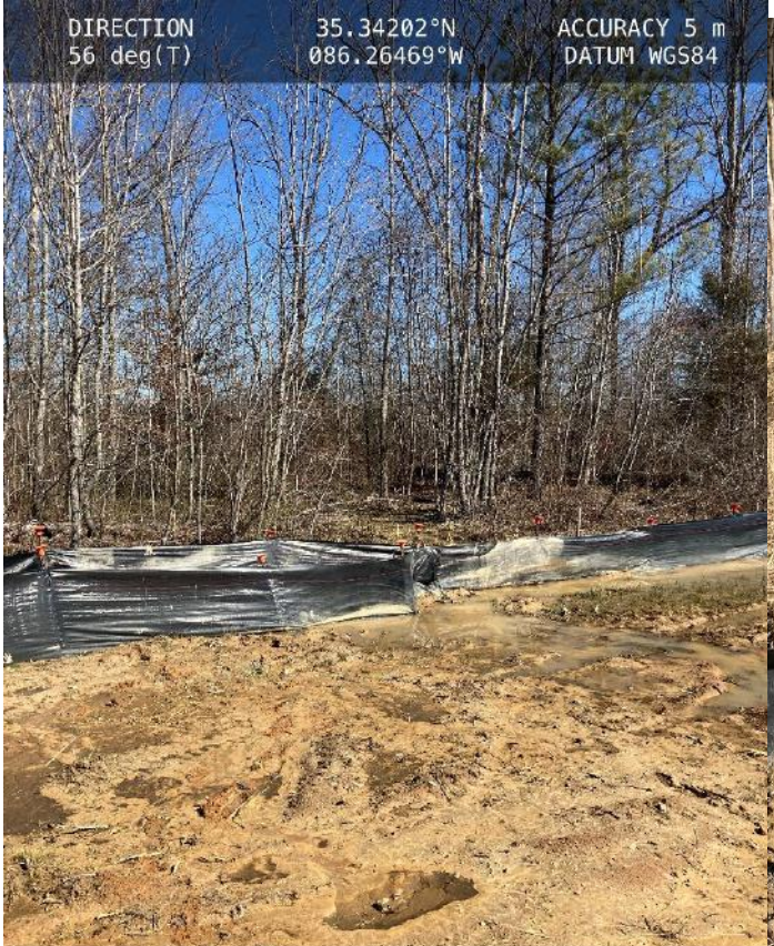
Zone 15 – Basin 34 Stabilize 2026-02-13 11:33:54-06:00
