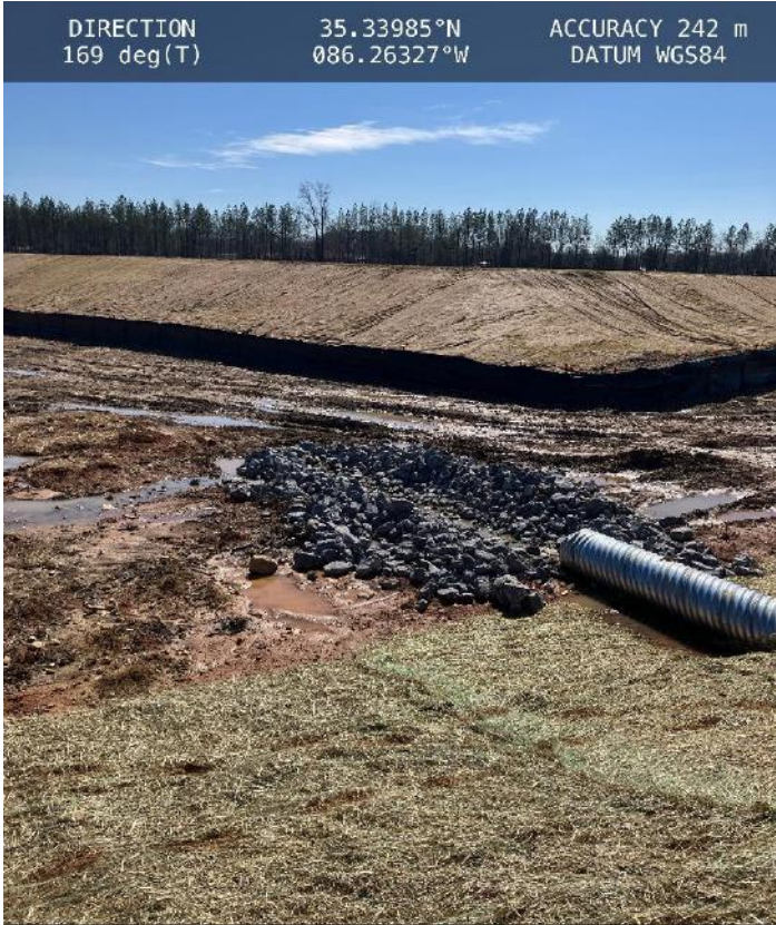
Zone 15 – Basin 34 Stabilize below outfall 2026-02-13 11:33:27-06:00
